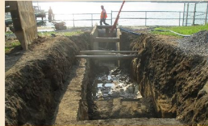
MILITARY WAREHOUSE FOUNDATION
