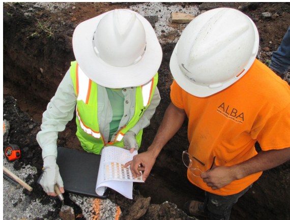
On site with my signature hard hat brim, showing the Munsell Color Chart to a crew member.
